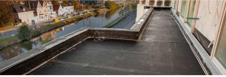
Besides the traditional flame welding of bitumen membranes, there are also many other ways to make a flat roof perfectly waterproof. When blowtorches are banned from the roof, roofers can apply the bitumen entirely without flame, using self-adhesive membranes, cold gluing or mechanically fixed systems. IKO offers the appropriate membrane or system for every one of these solutions. The overlaps in IKO roofing rolls can be welded with hot air or using an 'encapsulated flame'.
